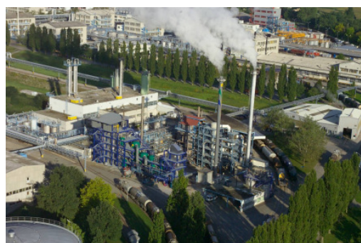
To achieve low emission values for particulates the flue gas treatment of the two incineration plants are equipped with Ring-Jet's
